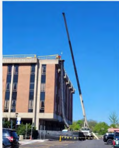
Ongoing New Roof Installation at LWH
