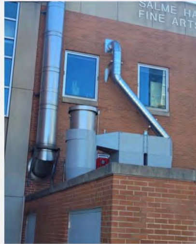
Fine Arts Dust Collector Project: Completion in the Summer '24
