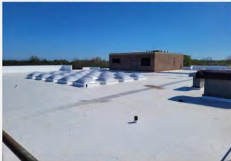
New Roof at BBH
