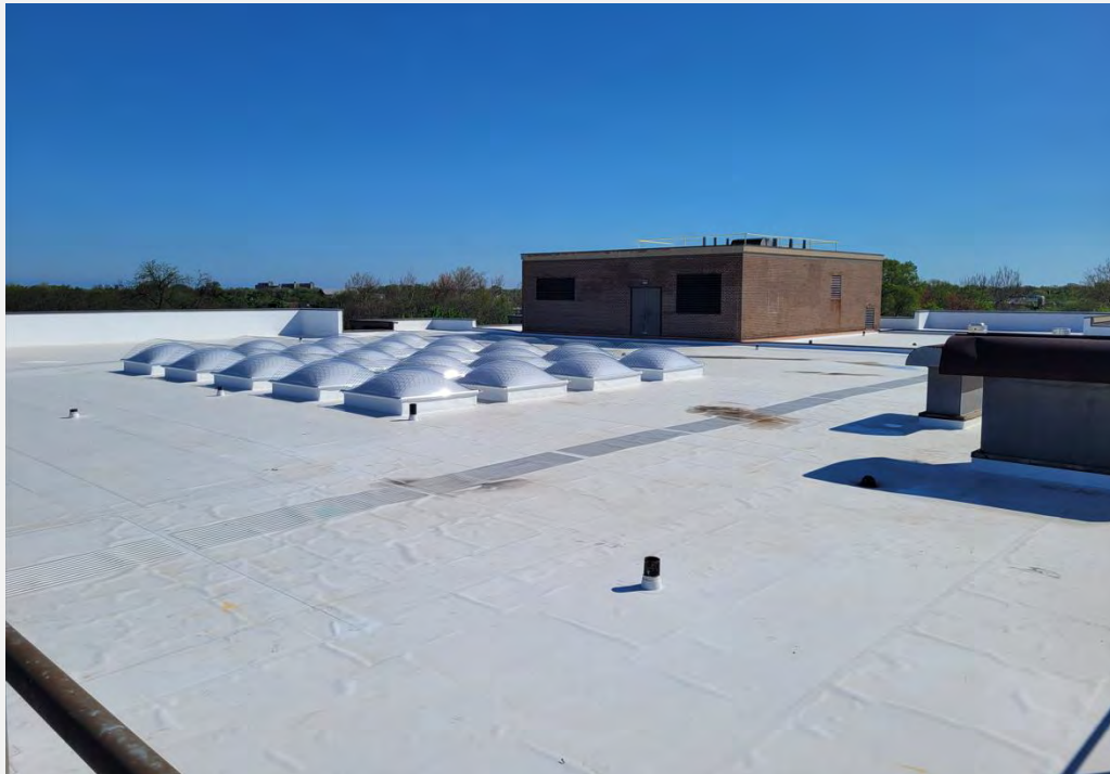
New Roof at BBH
