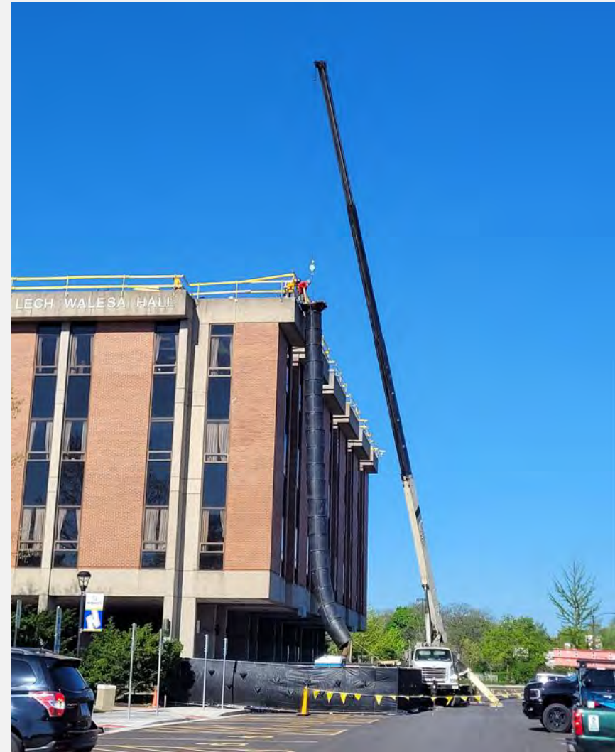
Ongoing New Roof Installation at LWH
