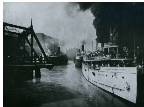
Chicago River at the Rush Street Bridge (1904).
